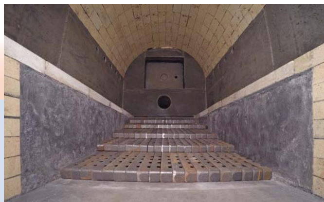
CAMERA COMBUSTIONE GRIGLIA MOBILE COMBUSTION CHAMBER MOVABLE GRILLE
